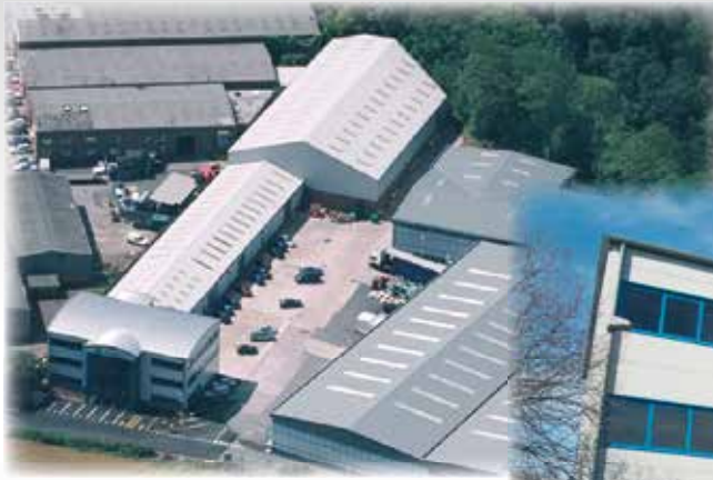
Cembre Ltd. factory in Curdworth (Birmingham)
