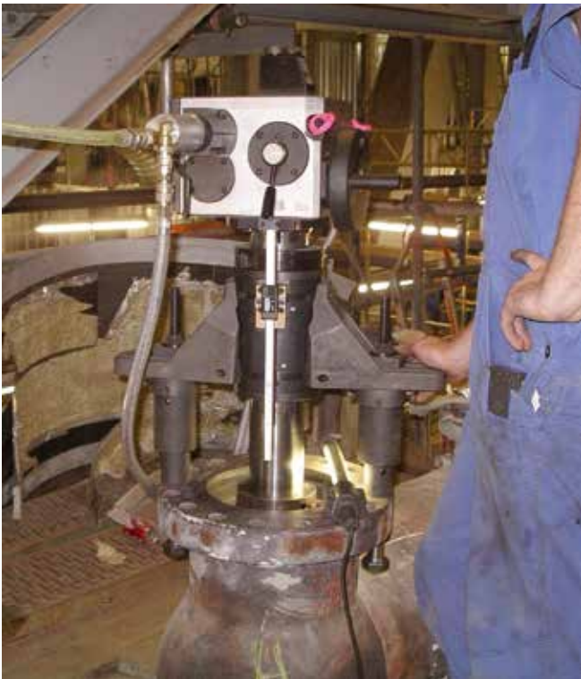
MD Application on site on a safety relief valve
