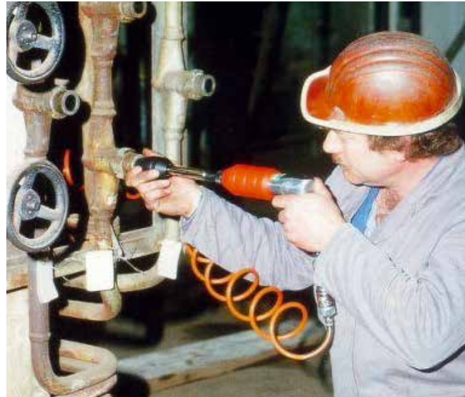
KVS grinding on-site
