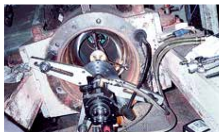
HTS 400 grinding on-site
