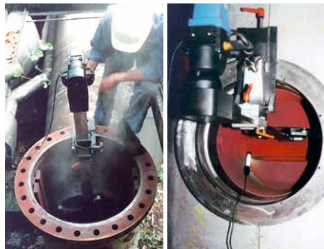
SHS 600 grinding on-site
